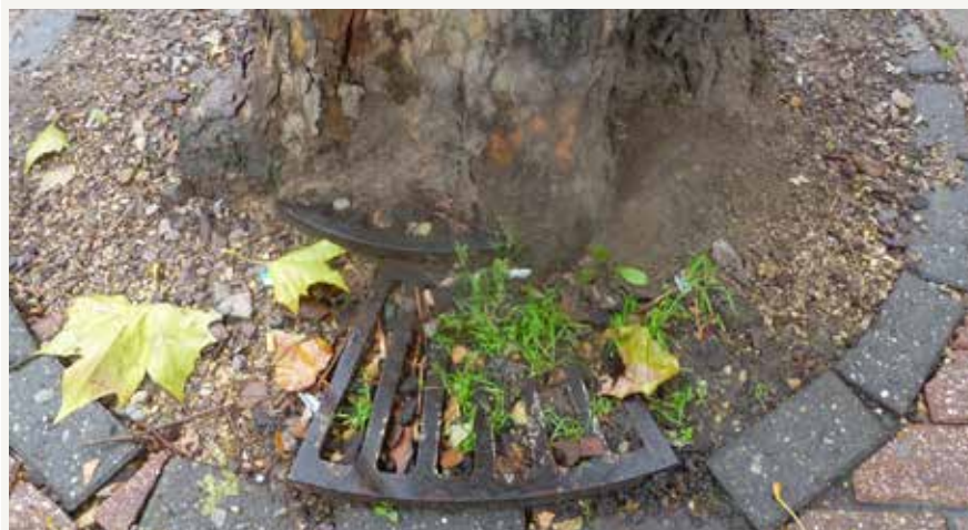
Bad aftercare: failure to remove this grille in time has caused permanent damage. © John Parker
