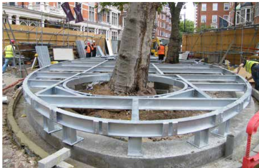
During construction: The Connaught Hotel, London. © Barrell Tree Consultancy
