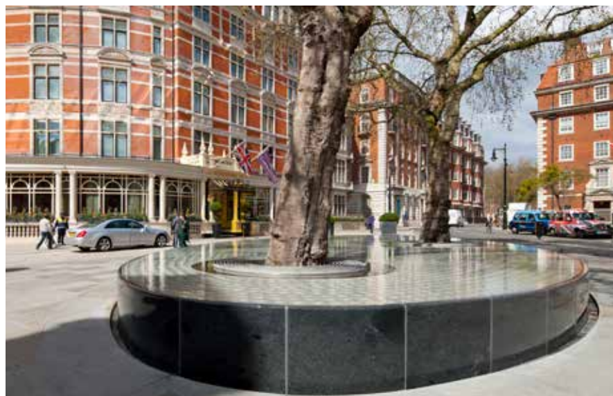
After construction: The Connaught Hotel, London. © Barrell Tree Consultancy
