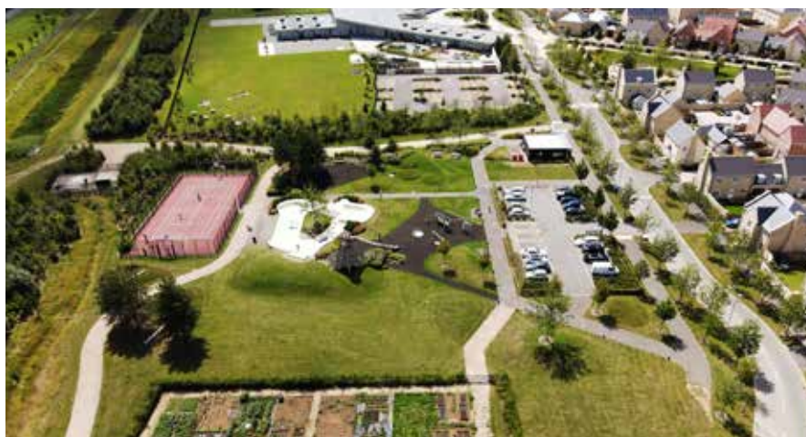
Investing in green infrastructure from the outset at Alconbury Weald. © Urban & Civic
