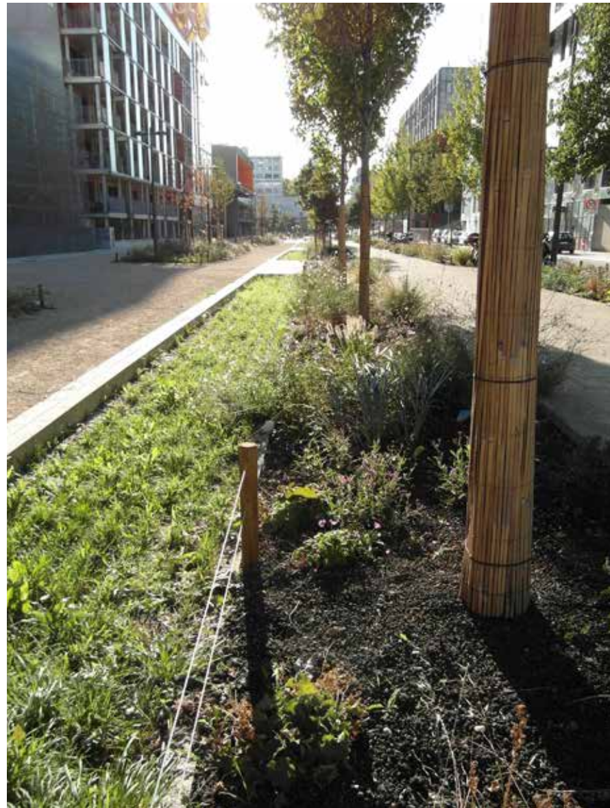
Trees play a critical role in managing surface water runoffs and enhancing biodiversity in the Lyon Confluence development. © TDAG
