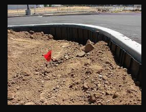
The theory is a simple one which suggests that tree roots can either be stopped from, or diverted away from, areas where tree roots cause damage to hard surfaces or building structures.
