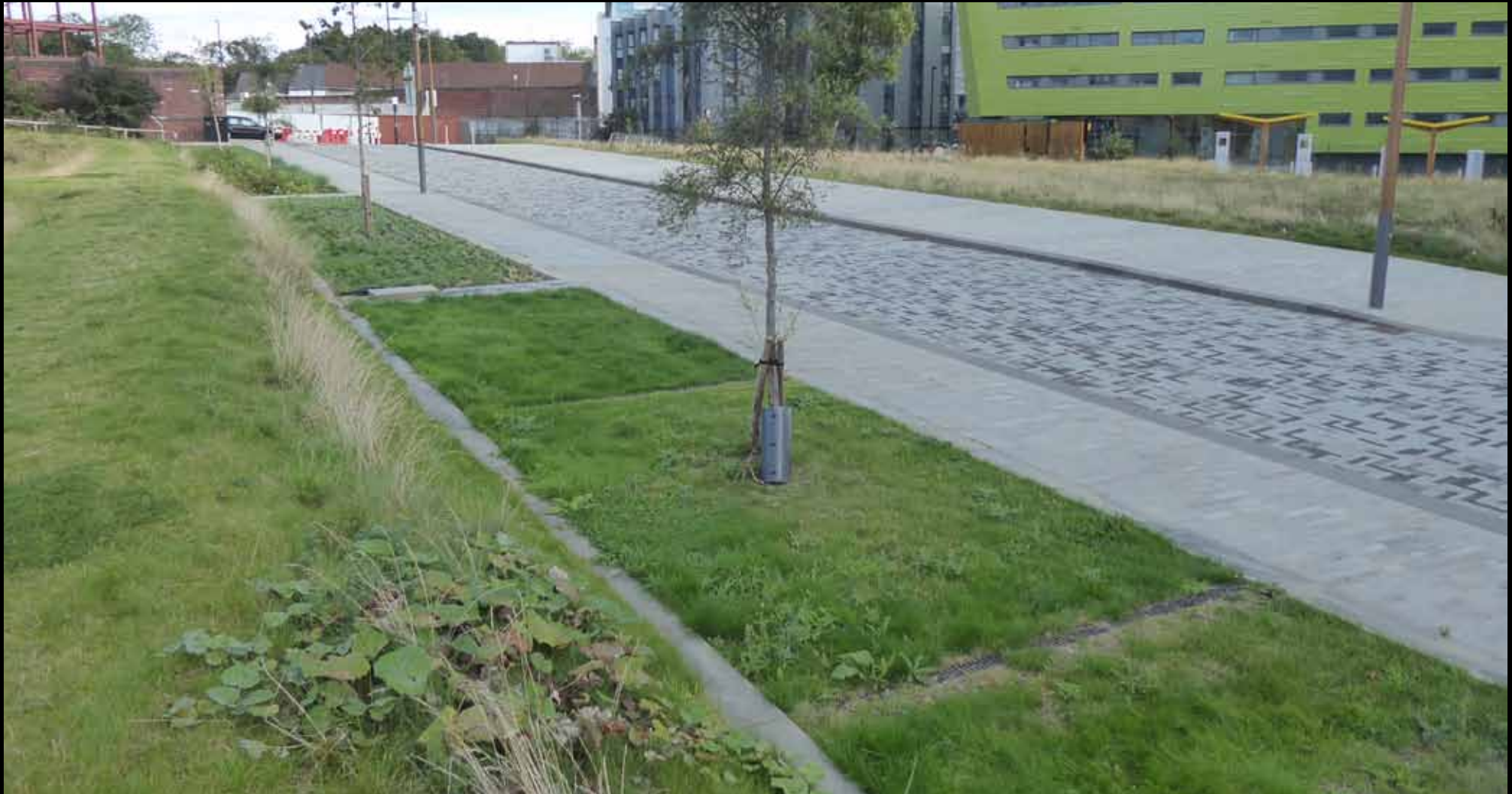
Green Infrastructure Facility, Newcastle University Science Campus
