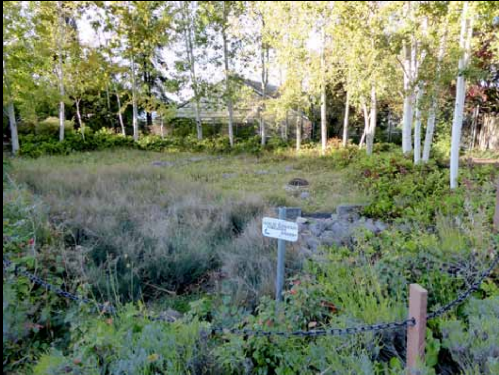
Glen Coe School SUDS, Portland , USA
