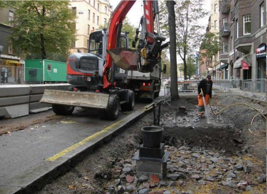
Flushing the soil into the structure
