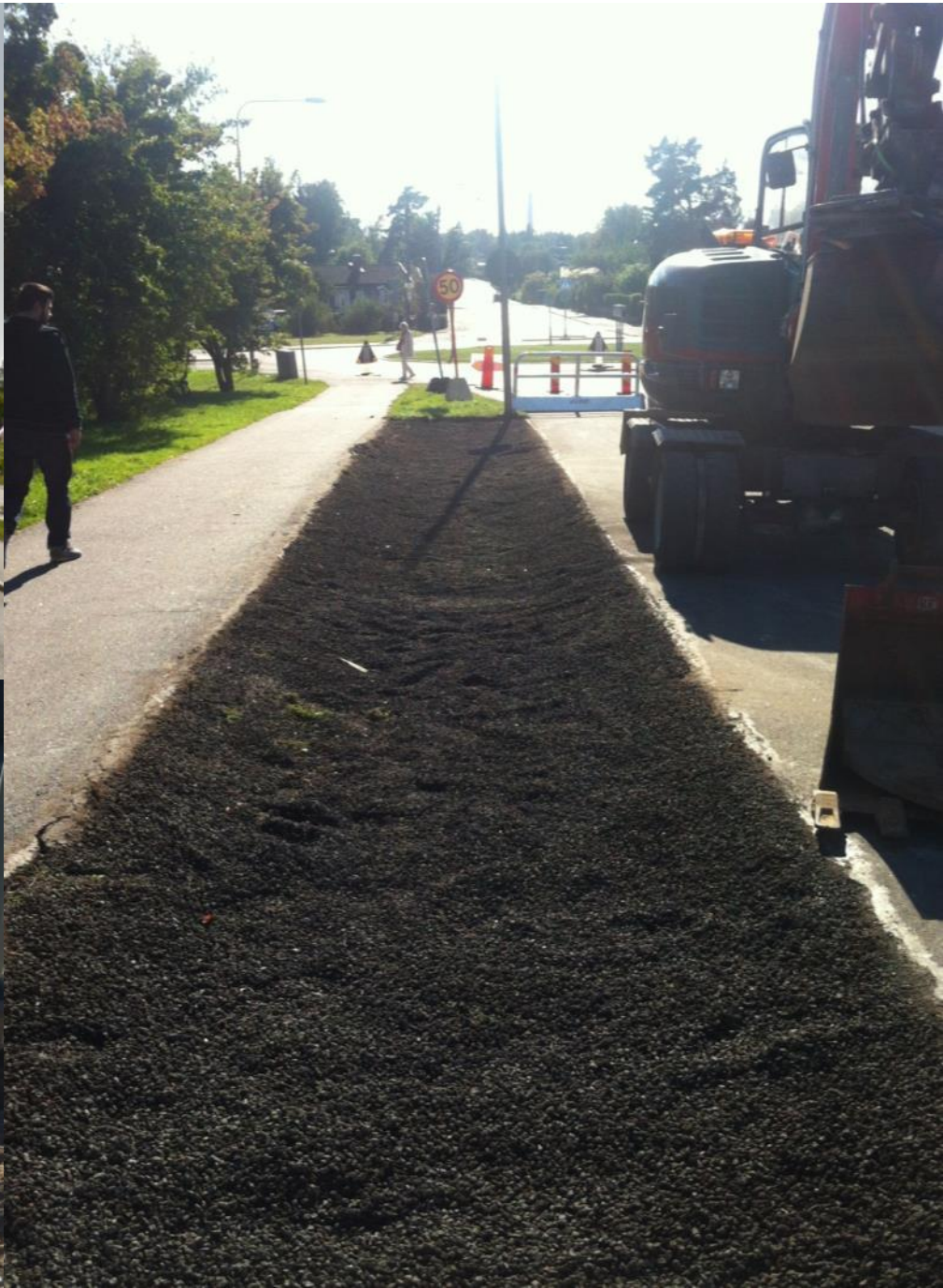
Plant bed for street trees charcoal macadam = crushed granite 8-16 mm mixed with nutrient-enriched charcoal
