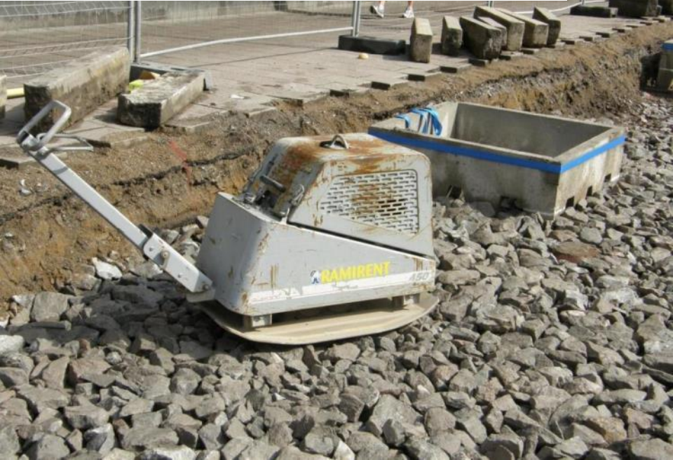
Compacting befor soil is washed in to the voids
