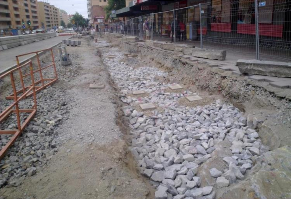
Compacting befor soil is washed in to the voids
