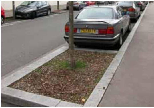
In a kerb buildout, woodchips provide a good surface opening treatment (Lyon, France). Image: Richard Barnes
