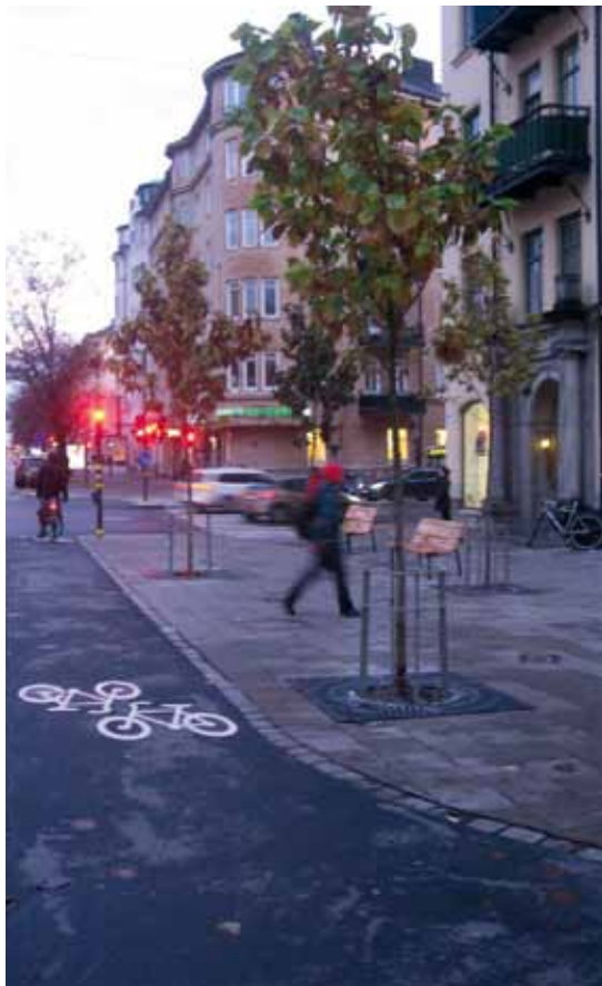
Low-level multipurpose protection in central Stockholm, Sweden
