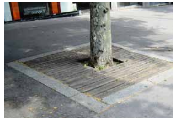
The opening of timber tree grates can easily be resized or tailored to accommodate trunk growth or mature trees (Lyon, France). Image: Frédéric Ségur
