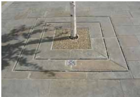
Grate with watering/aeration inlet and York stone infill matches surrounding paving at busy Dalston Junction bus station (Hackney, London)
