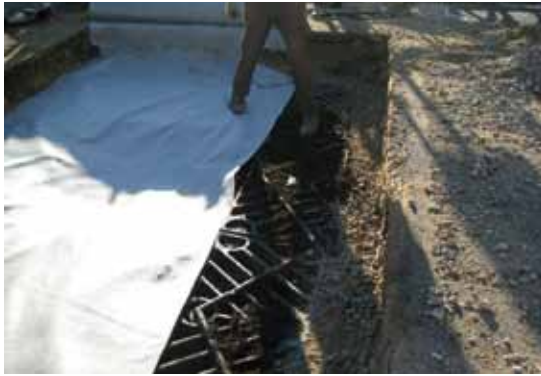
Placing the geotextile layer over the crates
