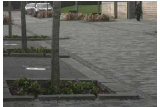
A low kerb and level drop protects the woodchip-covered tree surrounds from trespassing. Kerb opening ensures surface water runoff can flow in (Greenwich Peninsula, London)
