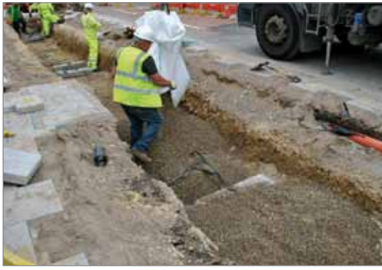
Drainage layer and root ball anchoring system
