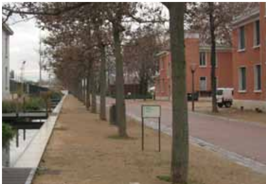
Self-binding aggregate used for roadsides in a new development (Lyon, France)
