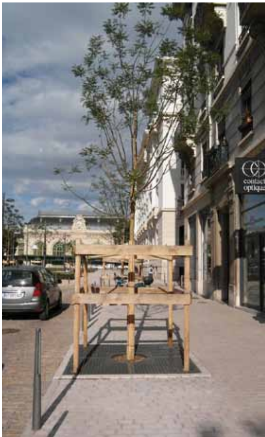
Bamboo mat and tree grate-mounted timber guard where greater protection needed in Lyon, France. Image: Sue James
