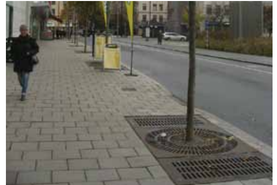
Extensive ductile cast iron grate facilitates water infiltration and effective gas exchange between above- and below-ground environments (Stockholm, Sweden)
