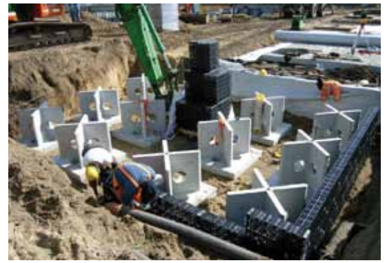
Placing cellular units around concrete crates
