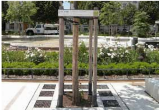
Tree grill with Limestone infill matches surroundings and facilitates water infiltration as well as gas exchange. Laid perpendicular to pedestrian flow to reduce slip risks (Place Bellecour, Lyon, France). Image: Sue James
