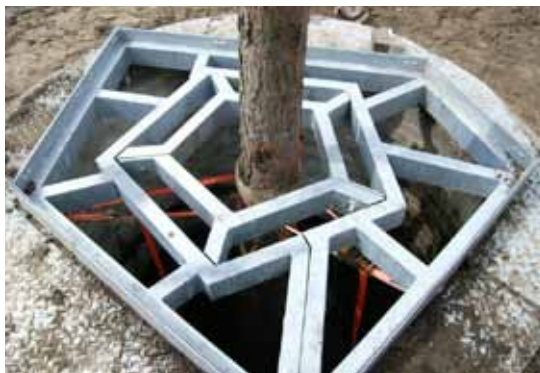
Substructure and completed conditions of the prominent bespoke tree grate installed at Apeldoorn Station Square (see Case study 22). Images: Ron van Raam (substructure), Jeremy Barrell (completed)
