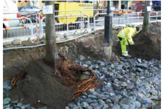
High quality soil is applied around the pruned/cleared root balls. Notice the root deformations caused by deep concrete casing used in the earlier planting hole design
