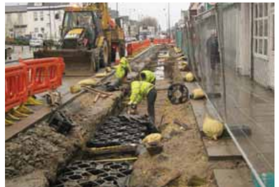
Compacting base and placing crates
