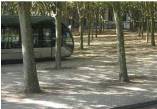
Continuous strips of self-binding aggregate between the footway and the tramway in Quinconces Square (Bordeaux, France)
