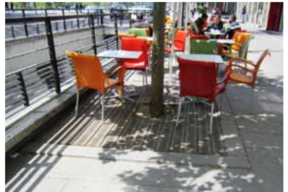
Non-slip timber tree grates provide a cost-effective and flexible solution. (Lyon, France). Image: Frédéric Ségur
