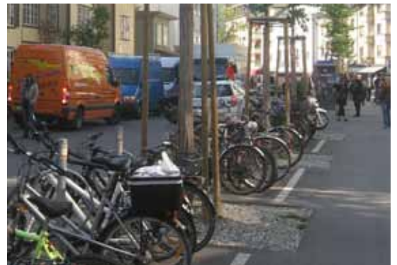
Simple loose gravel, laid slightly below the surrounding asphalt to avoid spilling (Bern, Switzerland)
