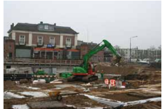
Filled islands topped with geotextile over a set of cellular units similar to those used around the installation. Protective covers are placed over planting holes
