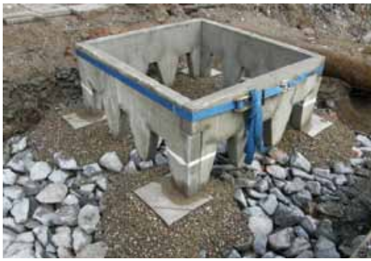
Positioning of concrete frame in continuous planting trench with large stones for skeleton soil along Hornsgatan, Stockholm (see Case study 25)
