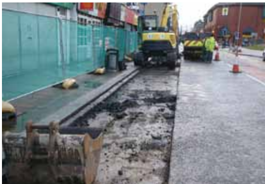
Excavation is starting along Ocean Road (see Case study 2)
