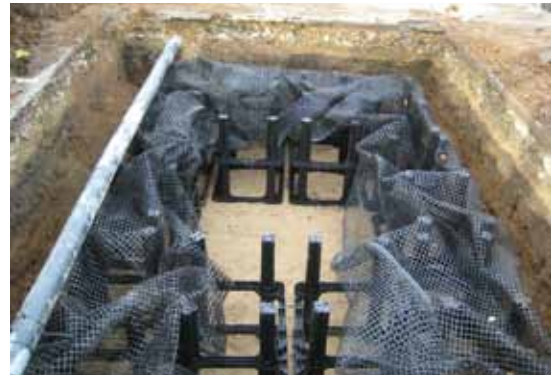
Placing the crates, accommodating the water main (see Case study 6)
