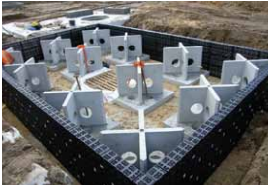
Ready for filling island with soil
