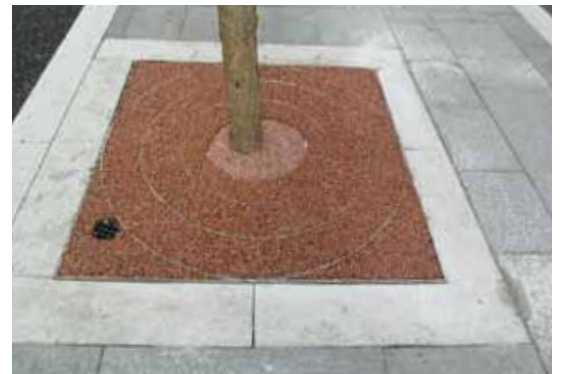
Grate with removable rings in resin-bound gravel and watering/aeration inlet on Swansea Boulevard (see Case study 17). Image: Sue James
