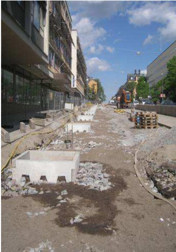
The whole of the pavement had been excavated to create a huge tree pit using large rocks and urban soil.
