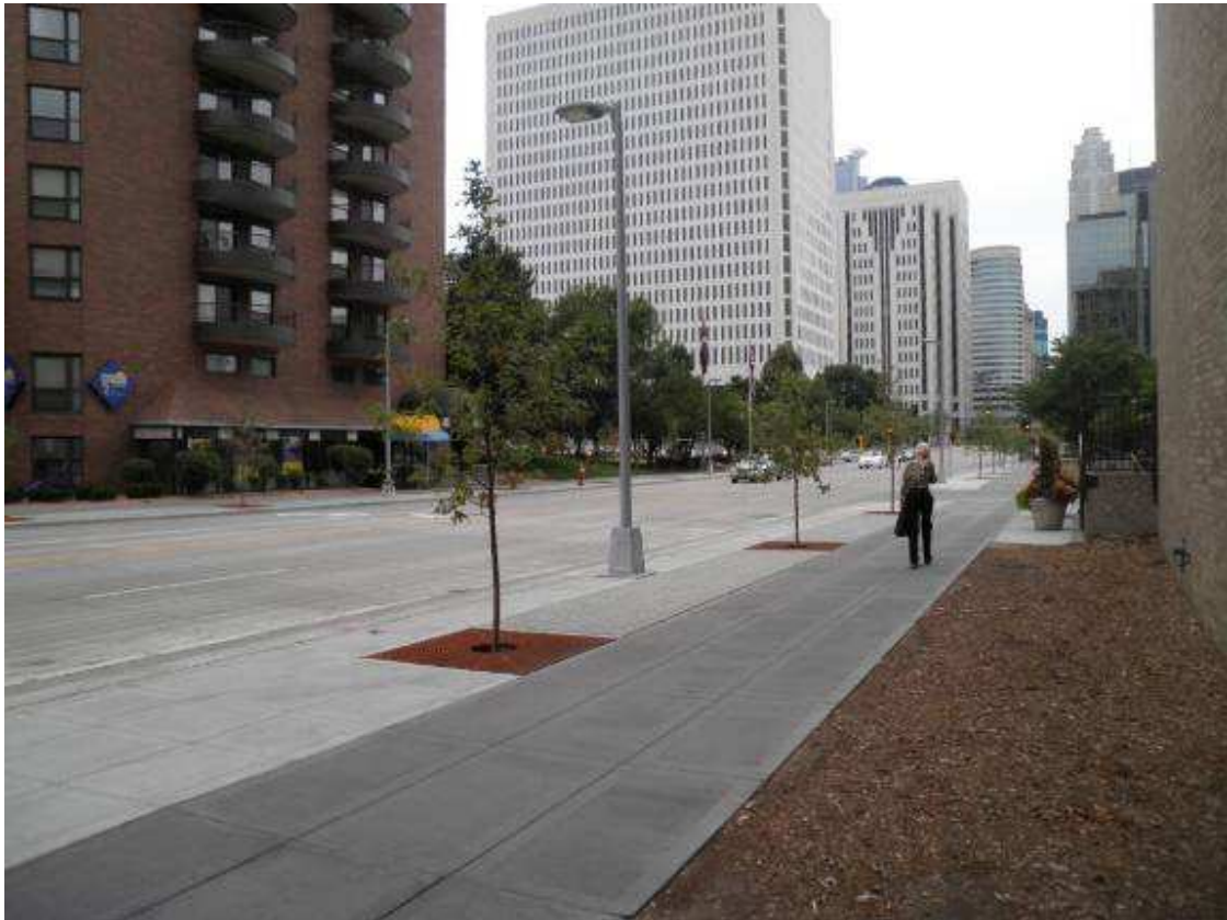
The linear crating systems provide 20 cubic meters of uncompacted soil per tree below the paving
