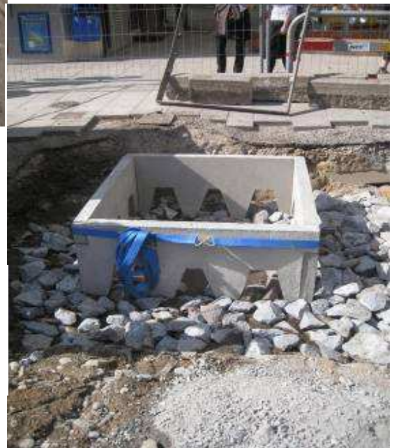
The trees are planted in cast concrete frames that deflect the tree root growth down below the construction detail of the pavement to the structured soil beneath.
