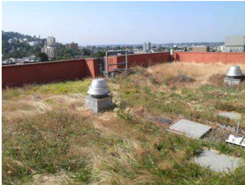
On average a roof garden retains approximately 50% of the rainfall on that roof
