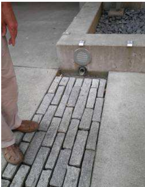
Innovative design transforms drainage into an attractive water feature
