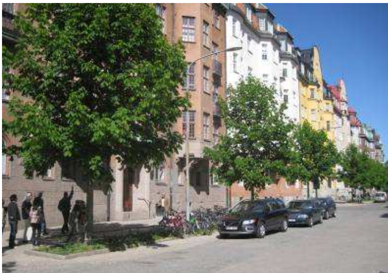
Erik Dahlbergsallen: Open topped trench with roof water feed
