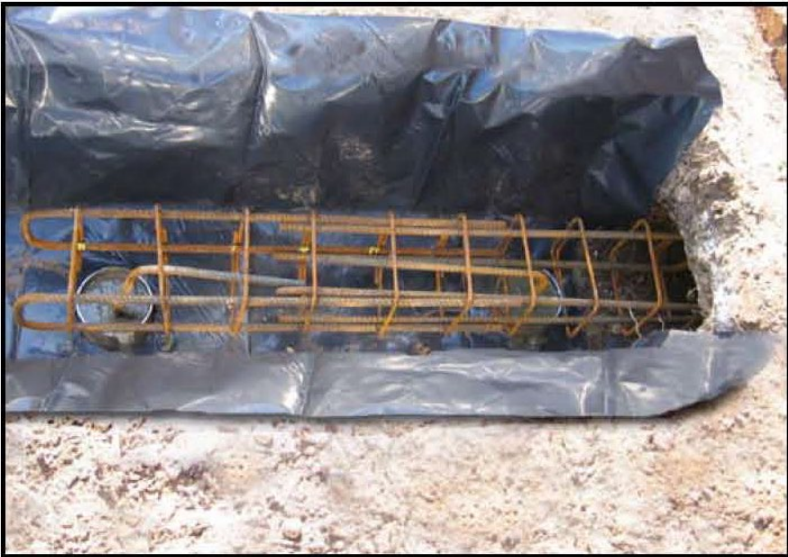
Piles completed - Beam steel reinforcement positioned
