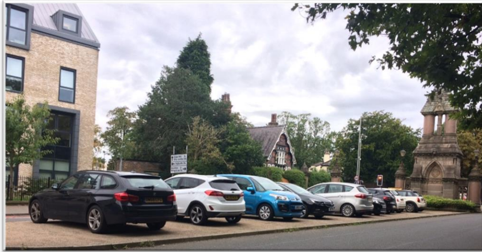
Removal of concrete 'parking' space
