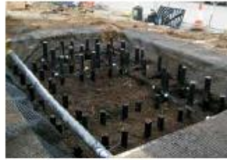
Filling the crates with tree soil.
