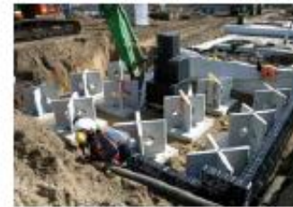
Placing cellular units around concrete crates.
