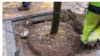
Compacting base and placing crates.
