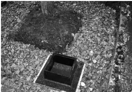
The aeration layer of smaller dry rock has been placed over the skeleton soil. It includes an aeration well, to be capped with a grate sitting flush with the paving.
