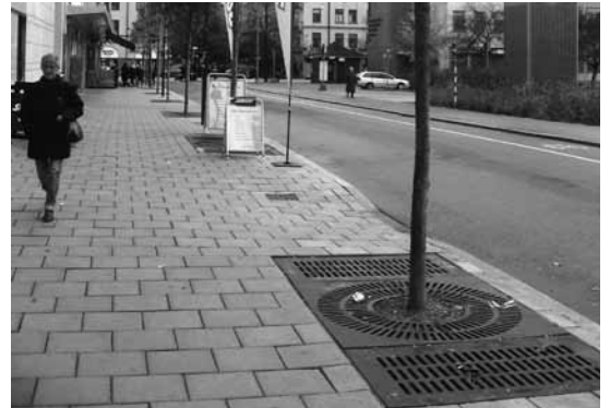
Extensive ductile cast iron grate facilitates water infiltration and effective gas exchange between above- and below-ground environments in Stockholm, Sweden.
