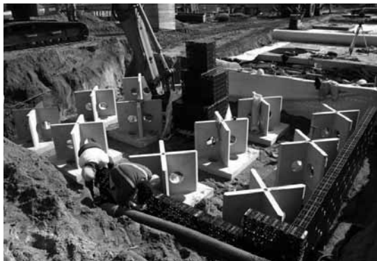
Placing cellular units around concrete crates.
