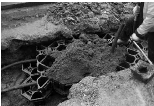
Crates with aeration/watering tubes being filled with soil.
