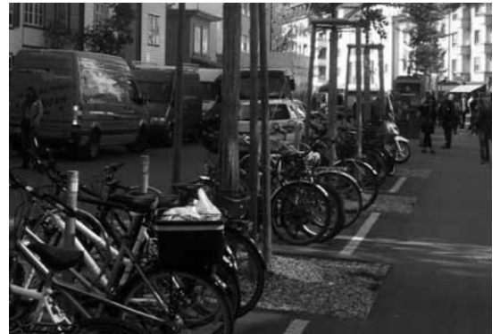
Simple loose gravel, laid slightly below the surrounding asphalt to avoid spilling in Bern, Switzerland.
