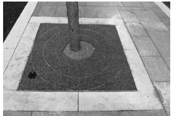
Grate with removable rings in resin-bound gravel and watering/aeration inlet on Swansea Boulevard (see Case study 17, p77). Image: Sue James
