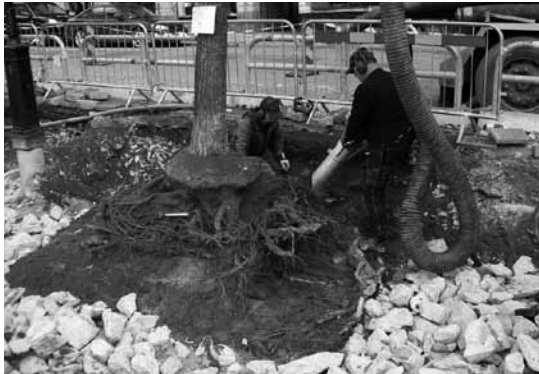
Some roots have been pruned. Excavation and soil clearing near the root ball is carefully conducted with non-invasive tool.
