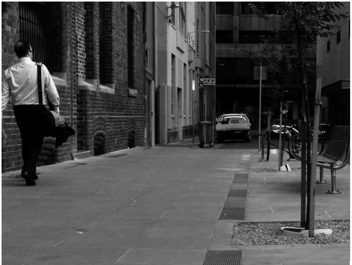
Infiltration trench directs footway surface water runoff to structural soil supporting the trees in Melbourne, Australia. Image: City of Melbourne
