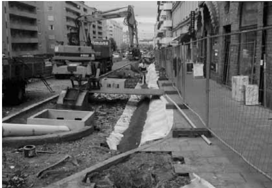
Utilities are being accommodated as part of the installation.
