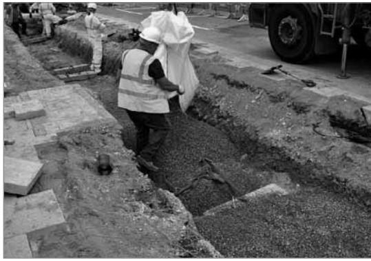
Drainage layer and root ball anchoring system.
