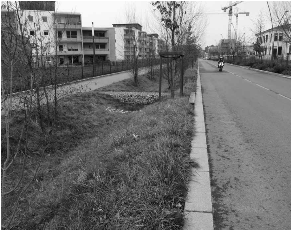
Swale between carriageway and footway in Sathonay near Lyon, France. Image: Richard Barnes
