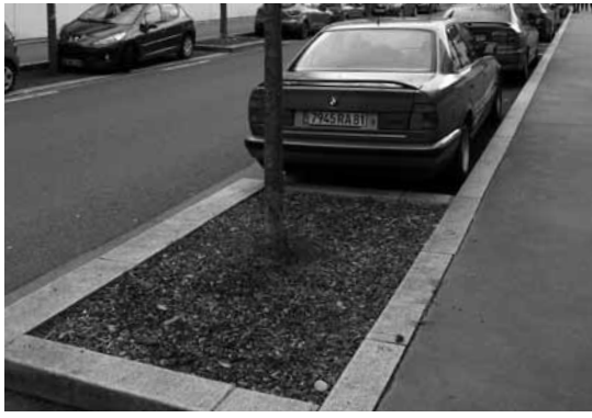
In a kerb buildout, woodchips provide a good surface opening treatment in Lyon, France. Image: Richard Barnes
