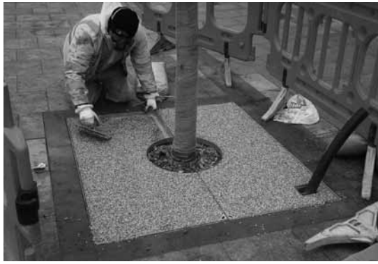
Grate with watering inlet and resin-bound infill and watering/aeration inlet on Ocean Road (see Case study 2, p31). Image: South Tyneside Council
