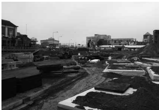
Filled islands topped with geotextile.
