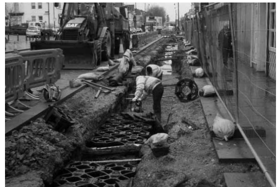
Compacting base and placing crates.
