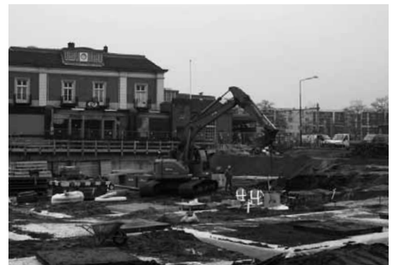
Protective covers are placed over planting holes.
