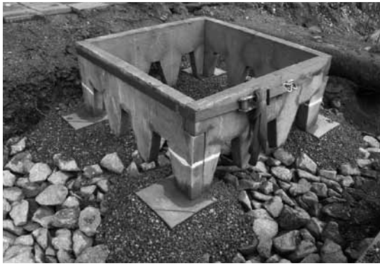
Positioning of concrete frame in continuous planting trench with large stones for skeleton soil along Hornsgatan, Stockholm (see Case study 25, p128).
