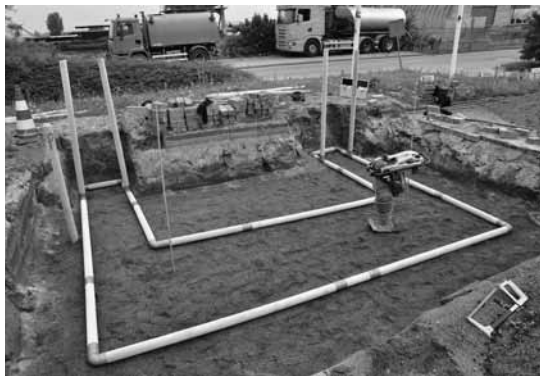
Site excavated and aeration system in place.
