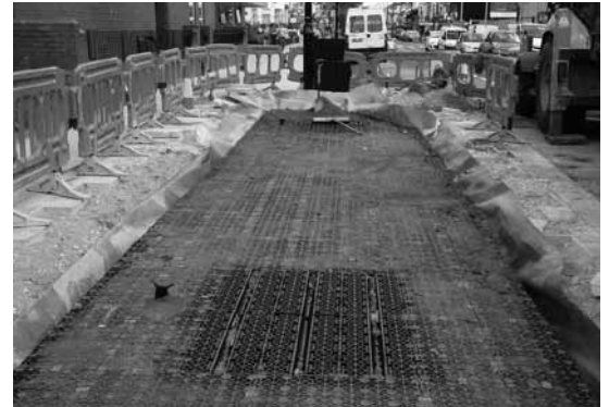
Permavoid units over geotextile membrane. Image: South Tyneside
