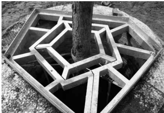
Substructure and completed conditions of the bespoke tree grate installed at Apeldoorn Station Square, The Netherlands (see Case study 24, p127). Images: Ron van Raam (left) and Jeremy Barrell (right)
