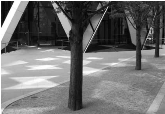
Well-maintained loose gravel provides porous surround for trees at 30 St Mary Axe, London. Image: Capita
