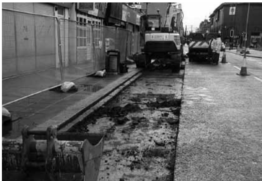
Excavation is starting along Ocean Road (see Case study 2, p31).
