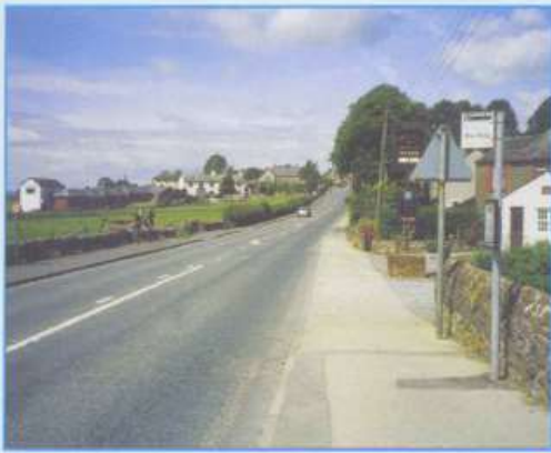
George and Dragon Pub before; and after, showing carriageway narrowing and planters
