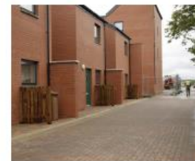
Hard edge to street Timber panels screen and protect wheelie bins
