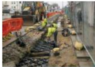
Compacting base and placing crates.
