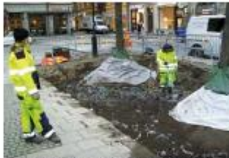
Root balls with new soil under protective cover and irrigation (notice the green watering bag around each tree). More soil is being flushed into the skeleton soil.
