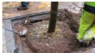
Compacting base and placing crates.
